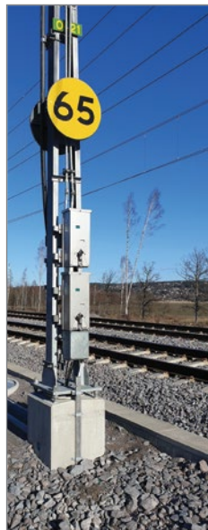
Dual installation of the motor operator Doppelte Installation des Motorantriebes
