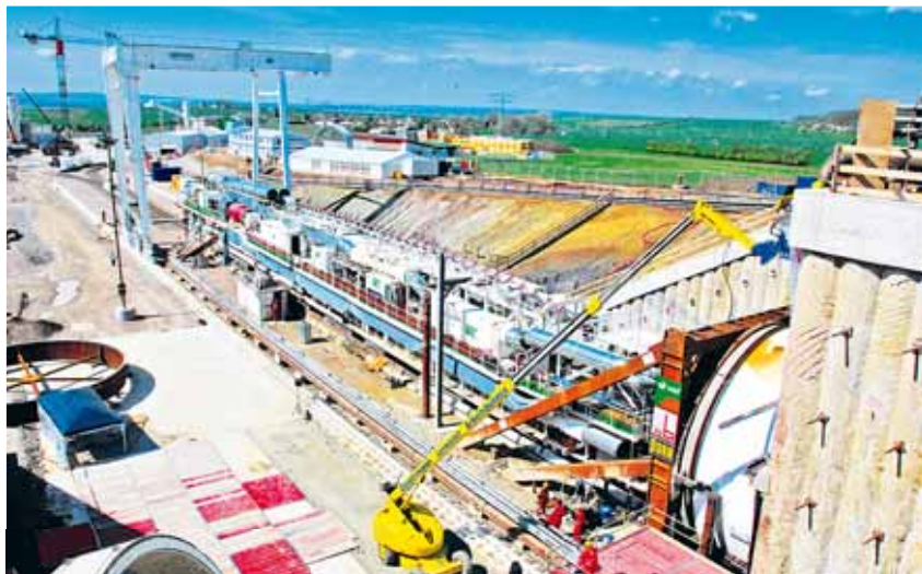
The TBM in the midst of the huge construction site.
