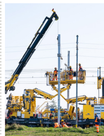
TSO train renewing overhead lines in the 1,500 volt network
