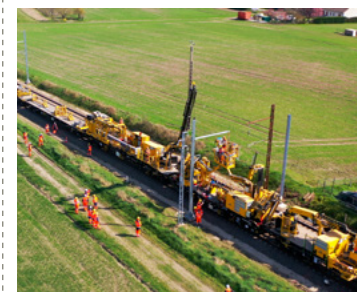
TSO high-capacity train in the 25-kilovolt network
