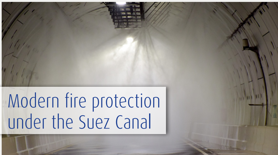
Acceptance test with spray test during commissioning
