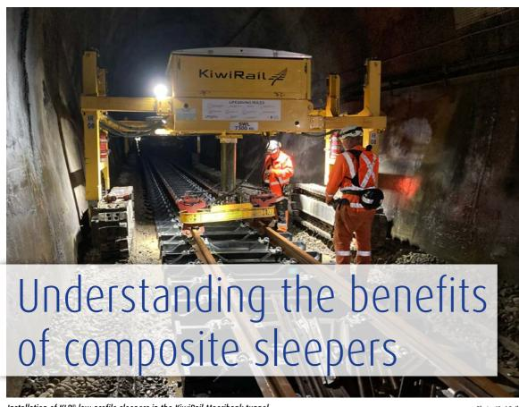
Installation of KLP® low-profile sleepers in the KiwiRail Maoribank tunnel.
